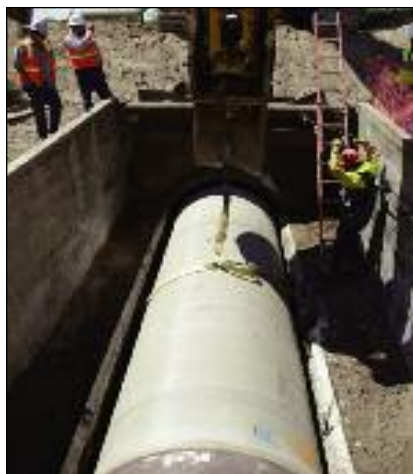
Figure 1 - 66" CCFRPM Hobas slipped into existing old 78" RCP
