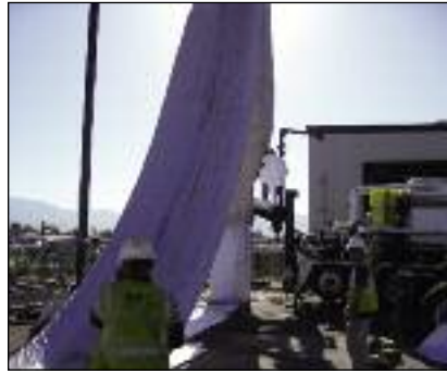
Figure 5 - 48" CIPP installed into existing 48" RCP
