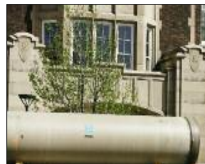
Figure 3 - 44" Hobas CCFRPM at job-site to be slipped into existing 48" RCP
