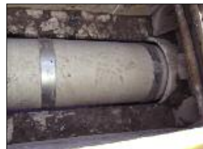
Figure 2 - CCFRPM Hobas Pipe with TeeKay Couplings at Insertion Pit
