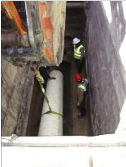
Figure 4 - 24" Vylon Pipe slipped into existing 27" RCP
