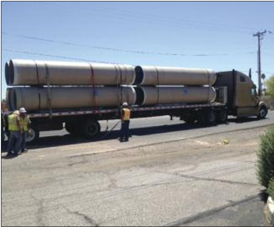
AUI sliplined 44-inch HOBAS Flush Relign pipe at Kirtland AFB.
