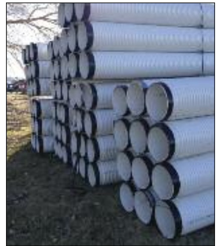
PVC liner pipe was used in an Albuquerque sewer line rehabilitation project.
